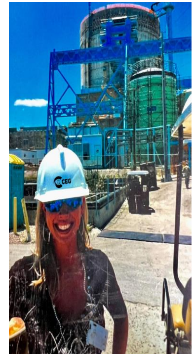
Turkey Point Nuclear Station Large Component Removal Project
