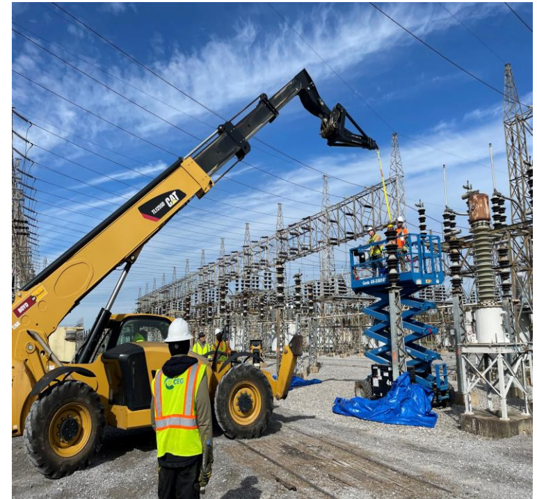
C537 Switchyard Project
