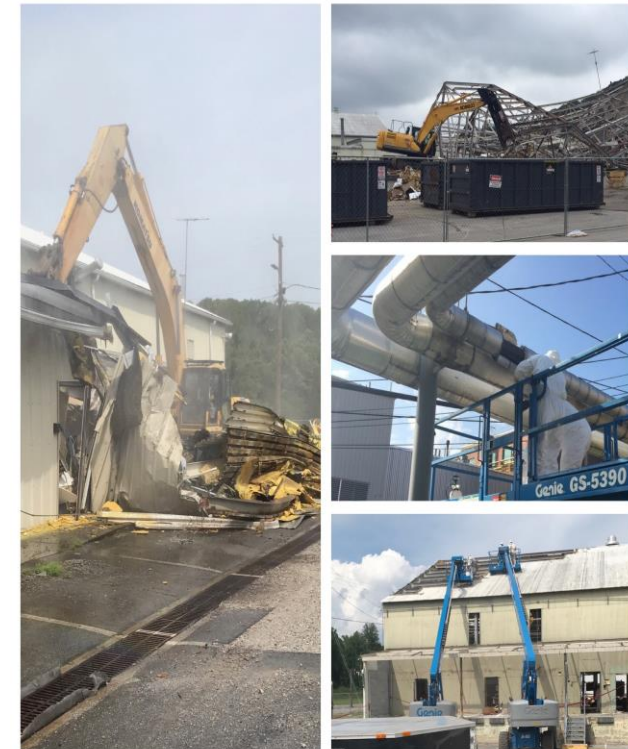
ORNL Building 7001 Radiological Demolition & ACM
