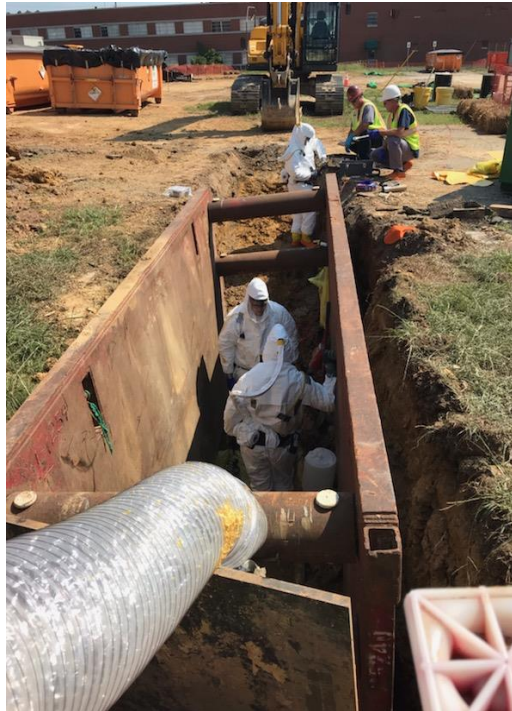
CEG Performed the First and Only Remediation and Removal of the Process Waste Lines and Liquid Low Level Waste Lines from the Original Hot Cells of the Manhattan Project at ORNL
